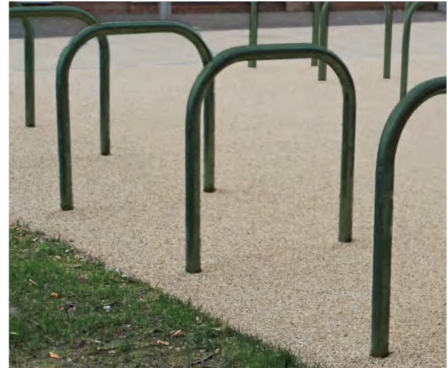
● Cycle stand, Sheffield style, dark green coating (TBC), root fixed. Located adjacent to welfare facilities.
