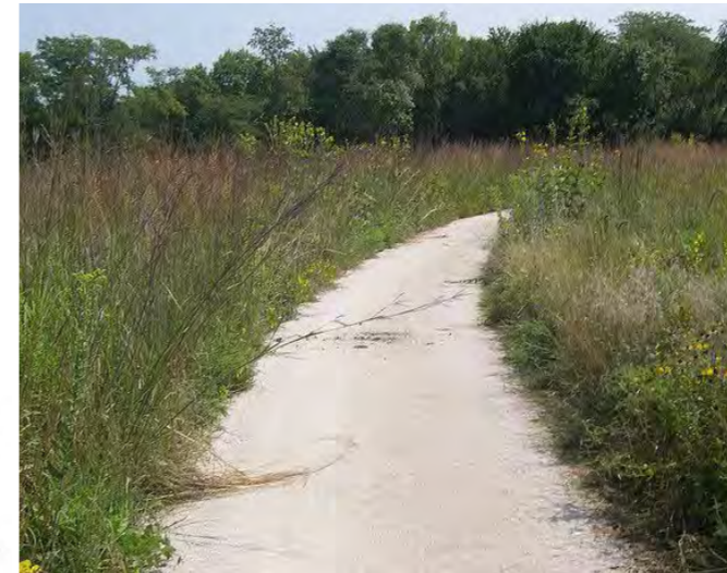
● Crushed limestone unbound paths - 2.4m wide
