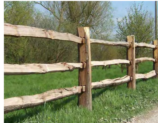
- - Traditional timber Cleft fence
