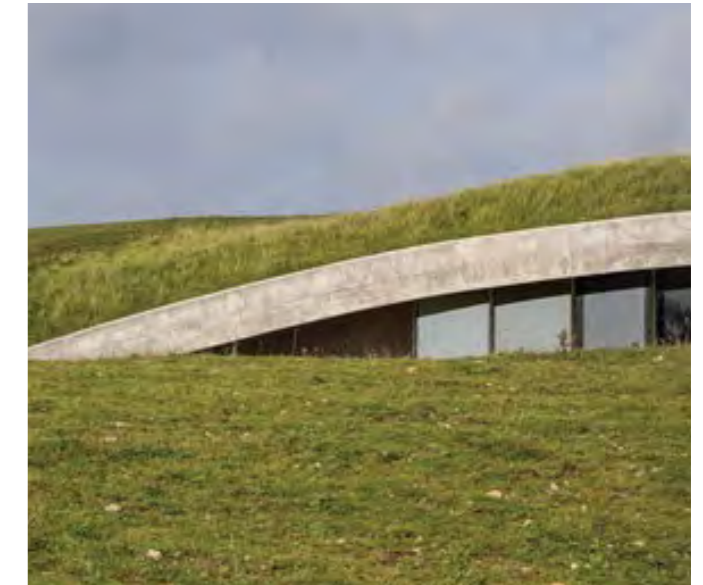
■ Proposed: Indicative - building embedded within chalk embankment with green roof for site welfare
