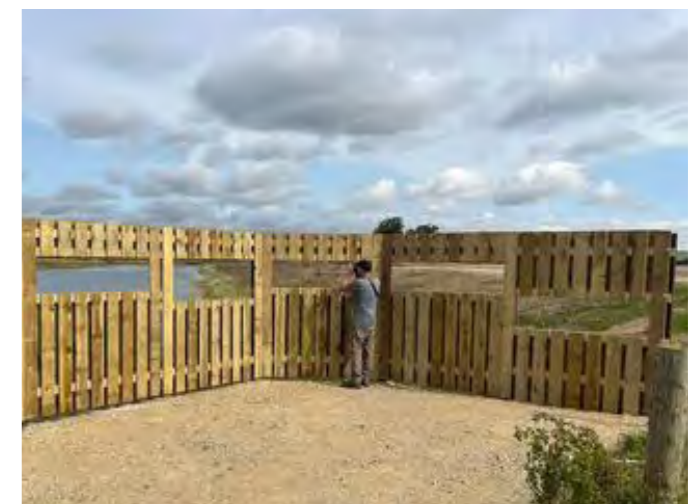
● Indicative: Timber bird hide screen/wall built into sloped bank to lake foreshore, nested within existing scrub planting
