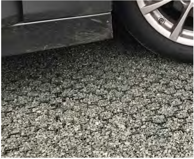
● Bodpave - Loose shingle within cellular confinement grid for parking bays.
