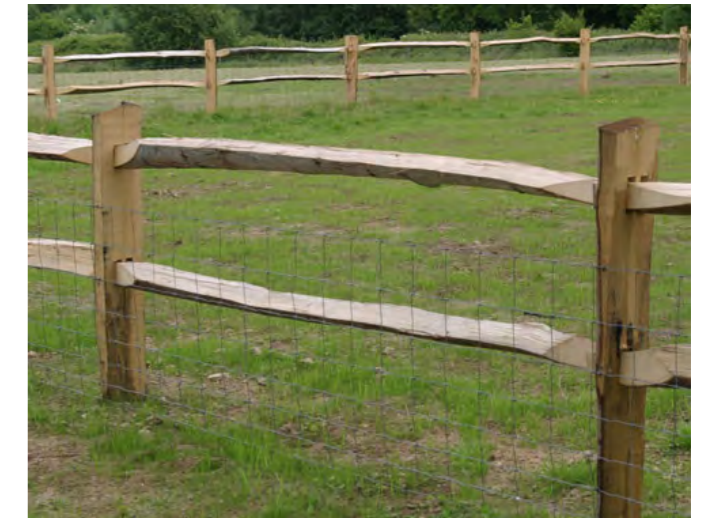
- - Timber Cleft fence with wire mesh panels where supporting grazing
