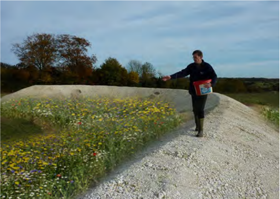
● Entrance feature: New landforms dressed with crushed chalk to both sides of the entrance road creating new site arrival and visibility screen to car park area
