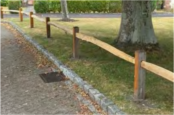
● Timber knee rails to protect ground flora
