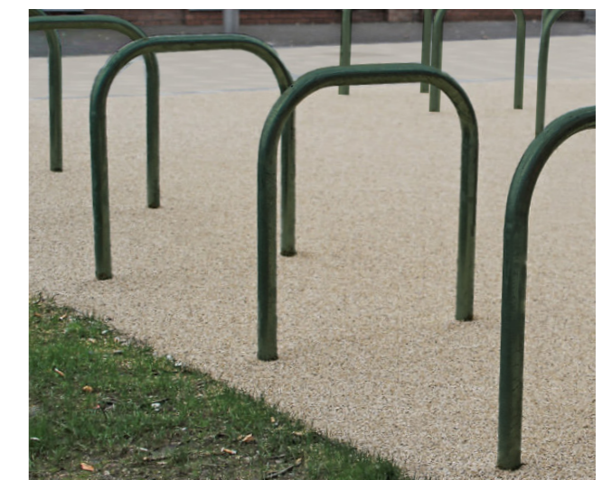
● Cycle stand, Sheffield style, dark green coating (TBC), root fixed. Located adjacent to welfare facilities.
